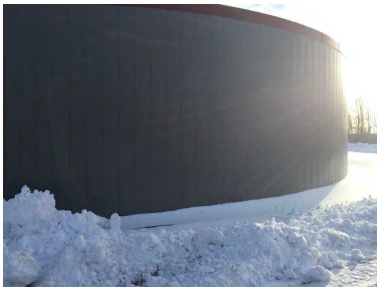
Figure 3.11: Second Stage Anaerobic Digester
