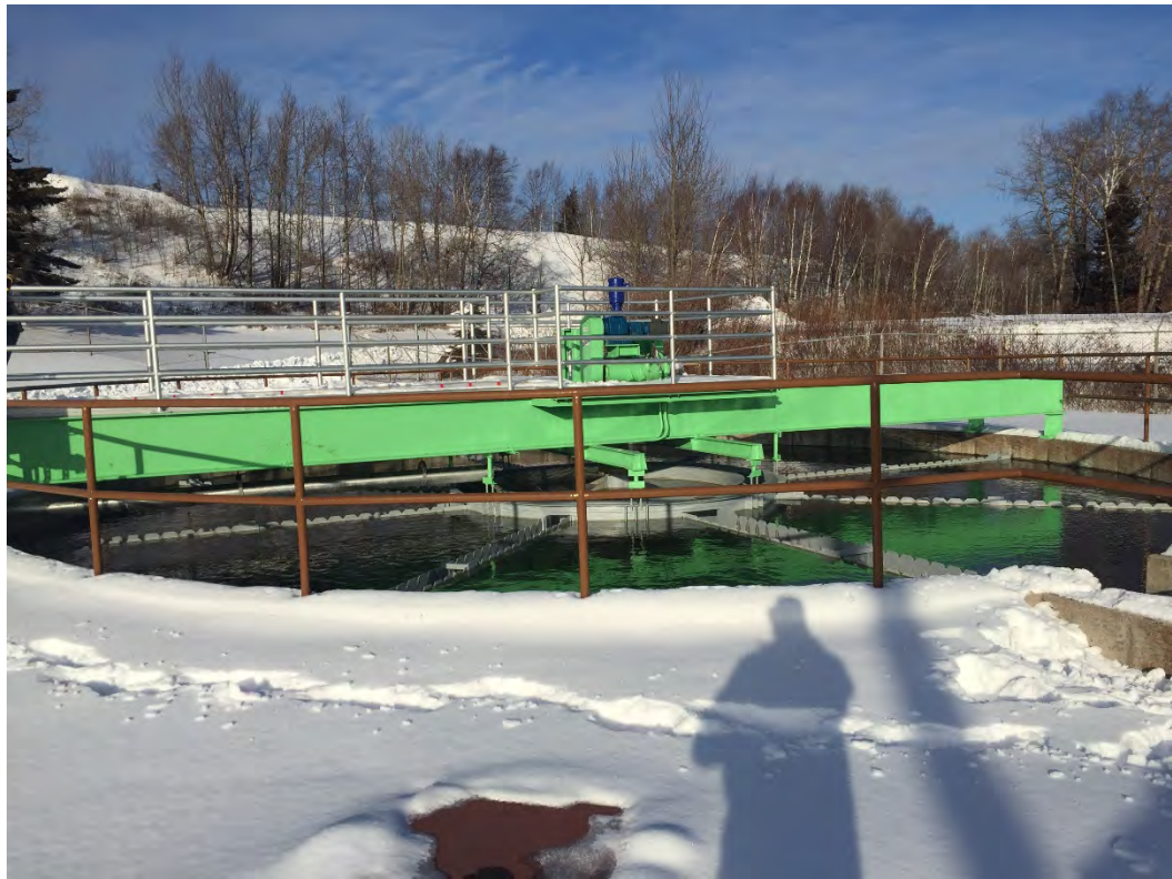
Figure 2.3: Solids Contact Clarifier No. 1
