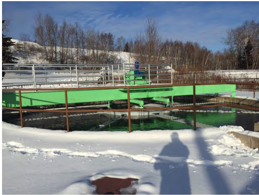
Figure 3.8: Solids Contact Clarifier No. 1
