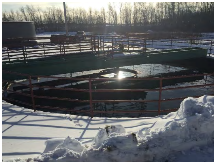
Figure 3.4: Primary Clarifier No. 2
