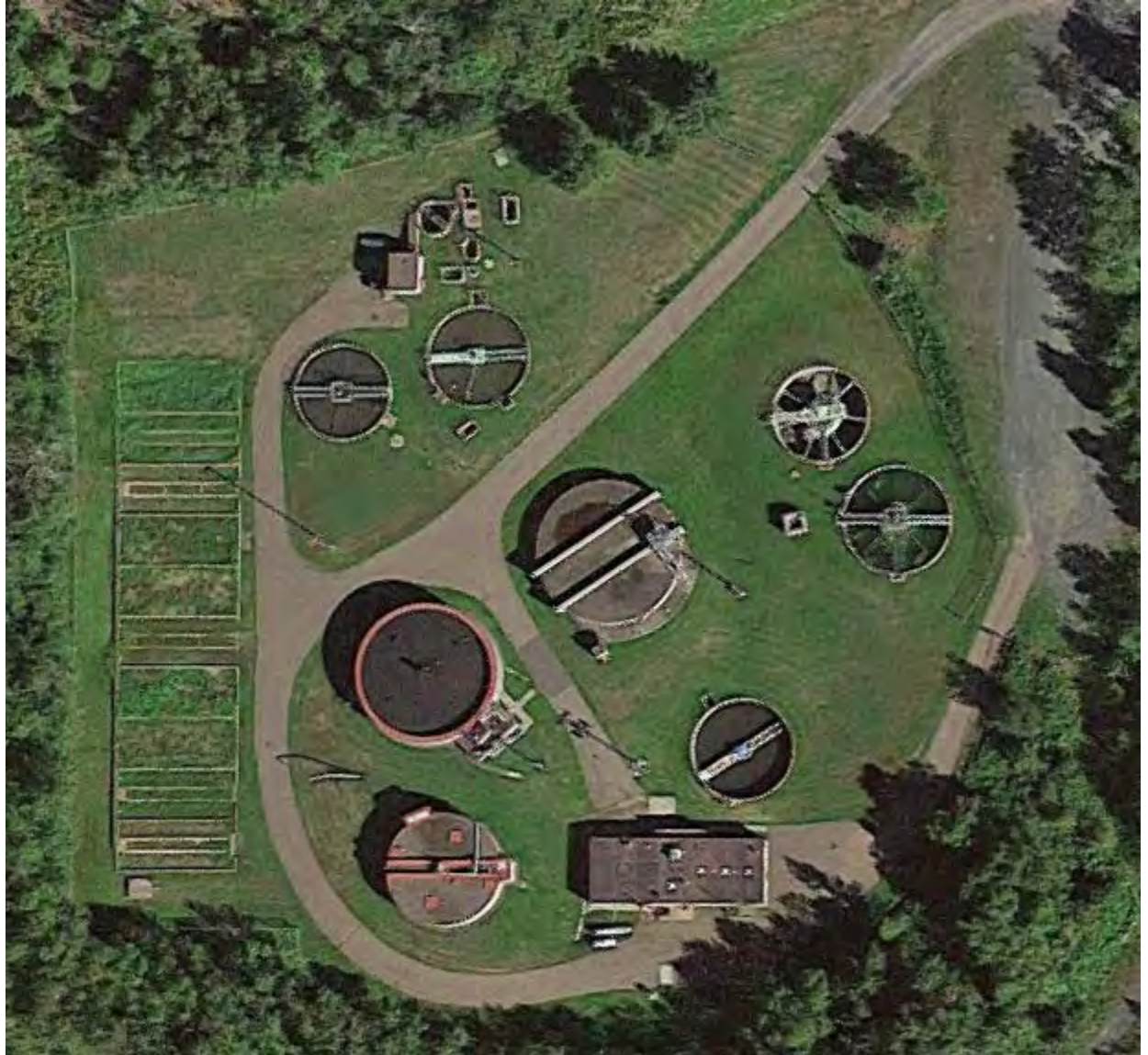
Figure 2.2: Aerial View of Silver Bay WWTF
