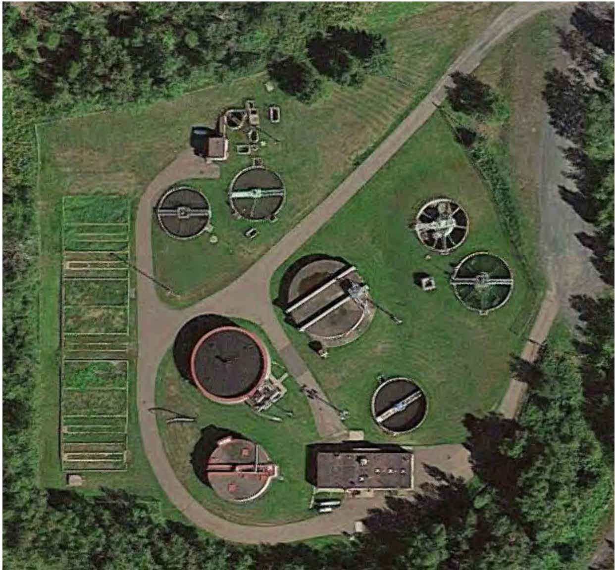
Figure 3.2 – Silver Bay WWTF Aerial Overview
