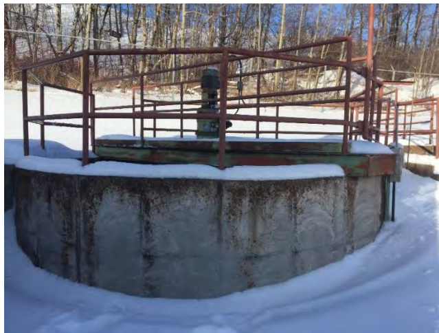
Figure 3.3: Grit Removal Chamber
