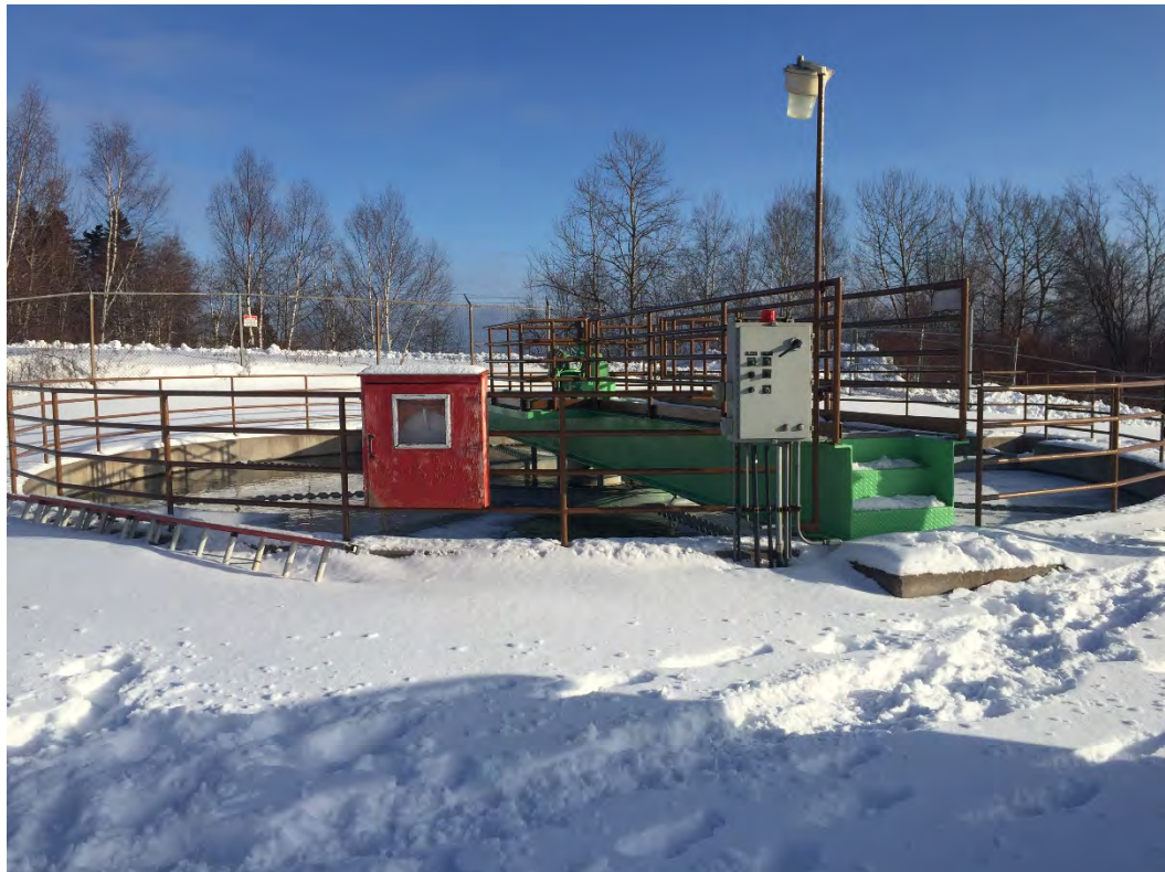
Figure 2.4: Solids Contact Clarifier No. 2
