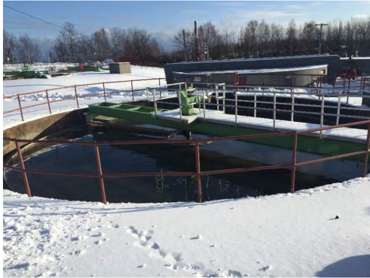
Figure 3.4: Primary Clarifier No. 1
