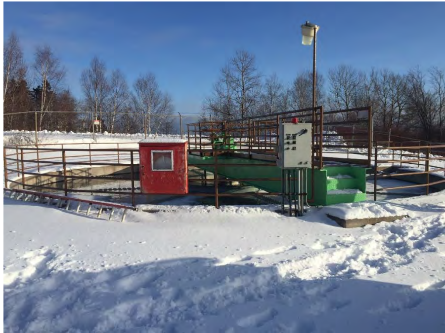
Figure 3.9: Solids Contact Clarifier No. 2
