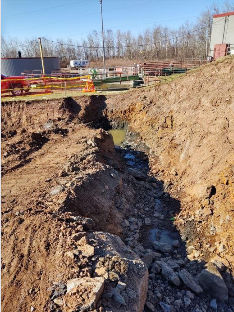
Pretreatment Building – Rock Excavation
