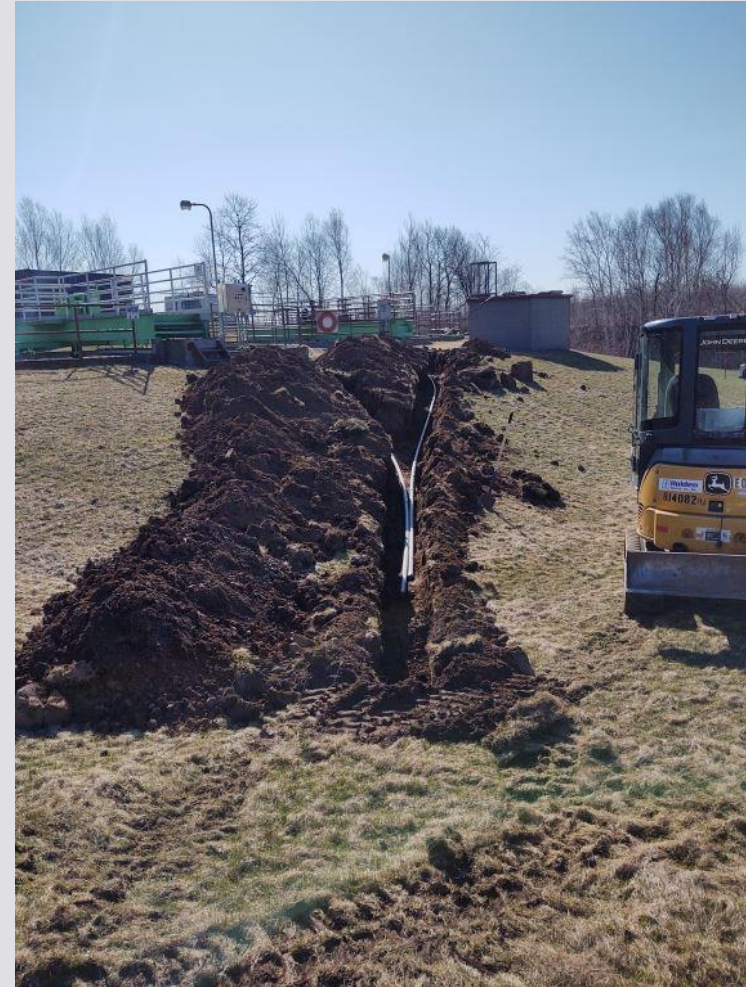
Pretreatment Building – Site Electrical Conduit Installation
