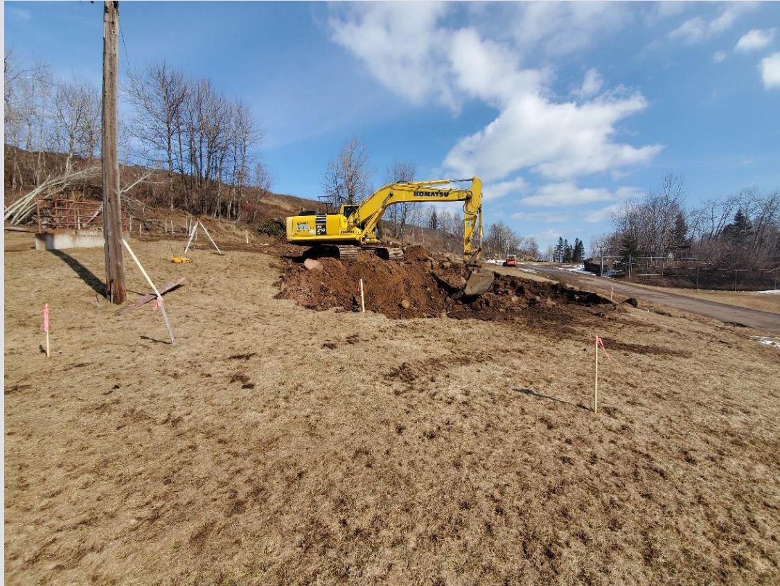
Pretreatment Building – Ground Breaking
