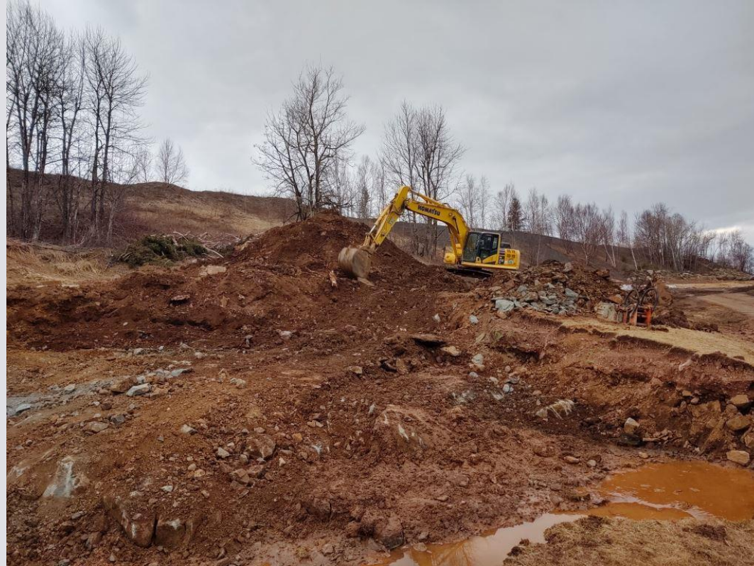
Pretreatment Building – Ground Breaking
