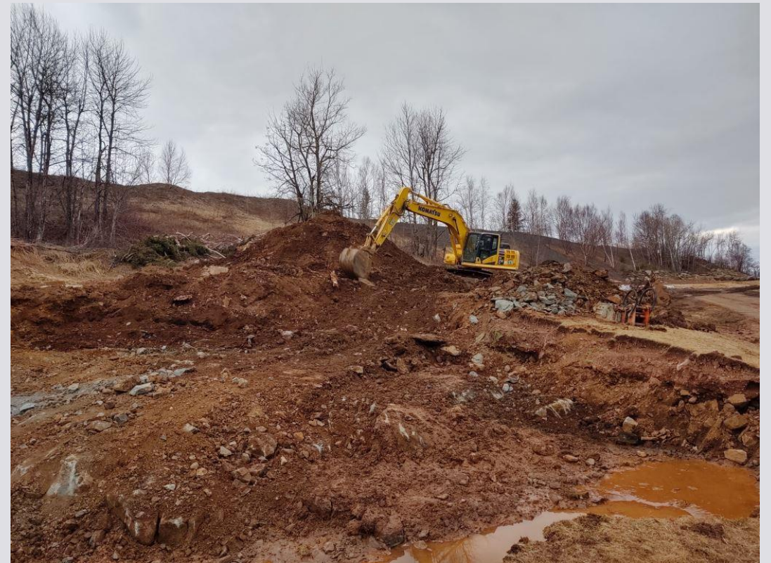
Pretreatment Building – Rock & Soil Excavation
