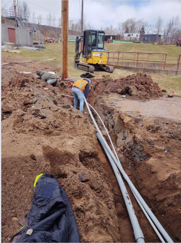
Pretreatment Building – Site Electrical Conduit Installation
