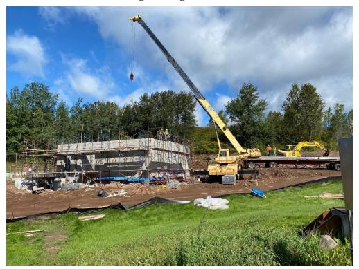
Pretreatment Building - With Finished Floor and Concrete Roof Plank
