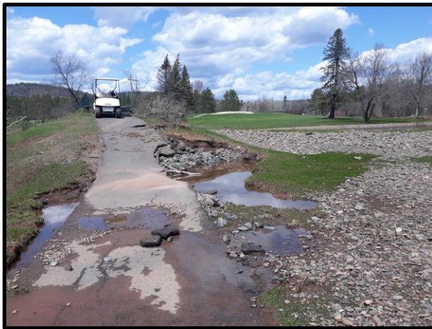
Photo 3: Damage to Cart Paths
